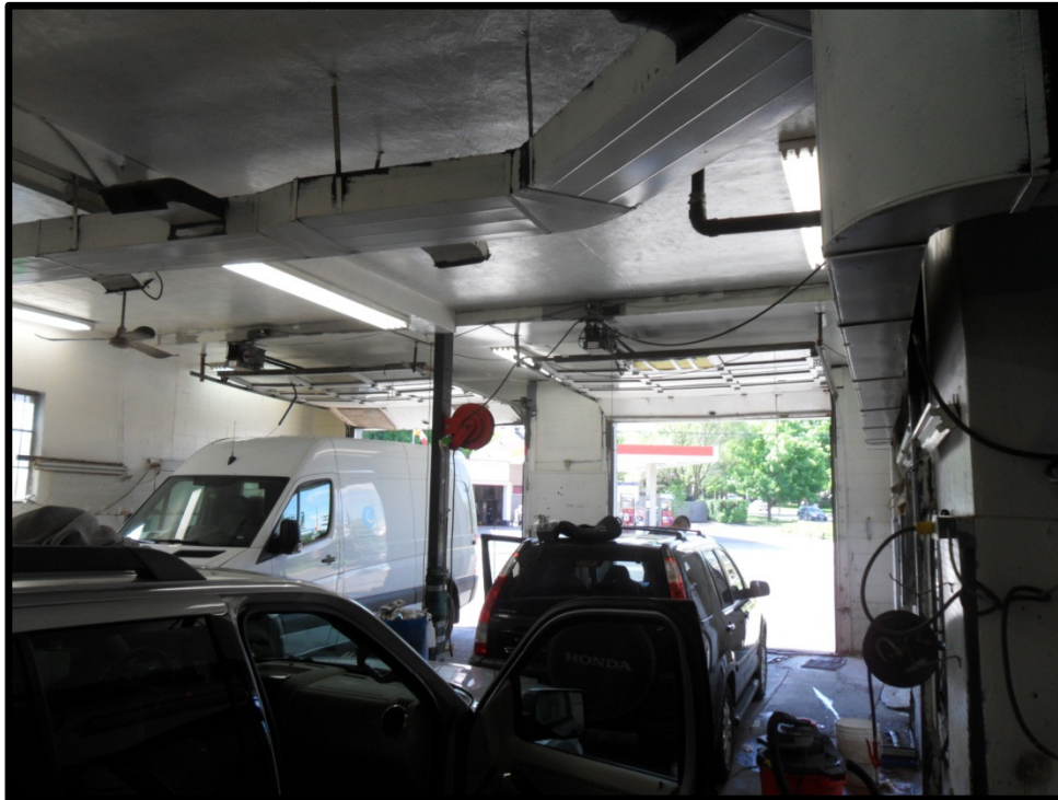
Photograph 5: View interior of eastern portion of the subject structure, looking south-southwest. Photograph illustrates carwash bays (former garage bays).
