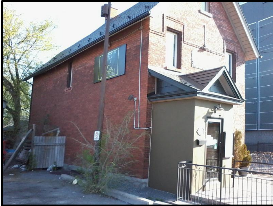
Photograph 11: Building at 1445 Wellington Street West, facing northeast.
