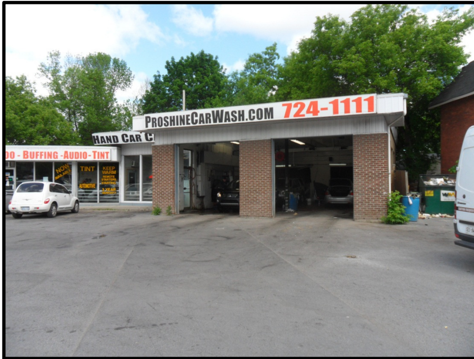
Photograph 1: View of the south side of the subject structure looking north. Photograph illustrates the location of the former automotive service garage as well as the water and sewer services (cut in asphalt).
