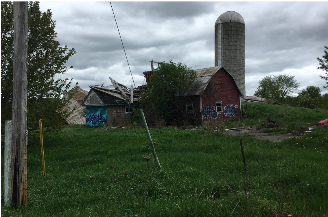
Photograph 8: View of the abandoned farm buildings.
