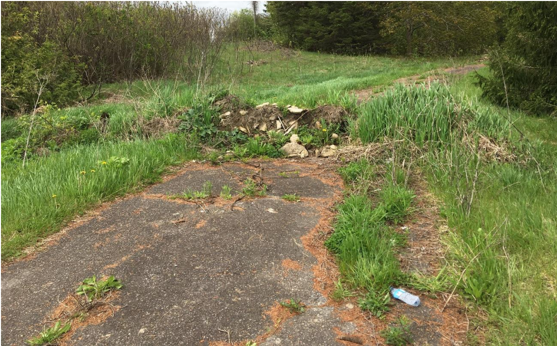
Photograph 1. View of the property entrance, looking south.
