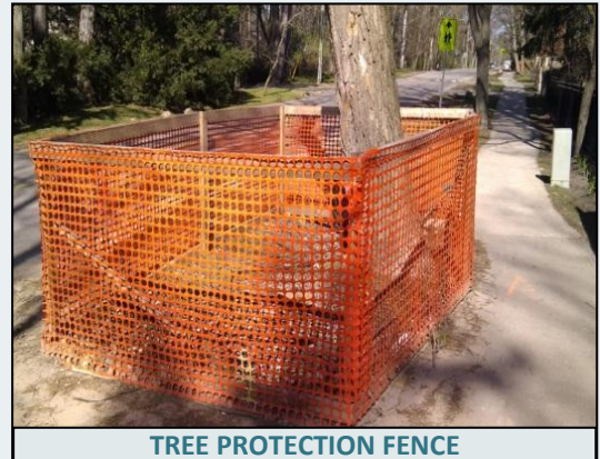
TREE PROTECTION FENCE
