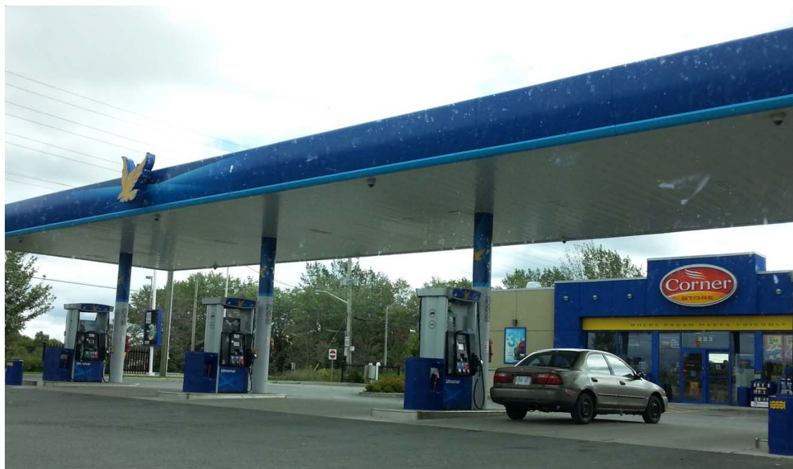
Photograph 14: Gas Station and convenience store located northwest of the Site, within the Study Area.
