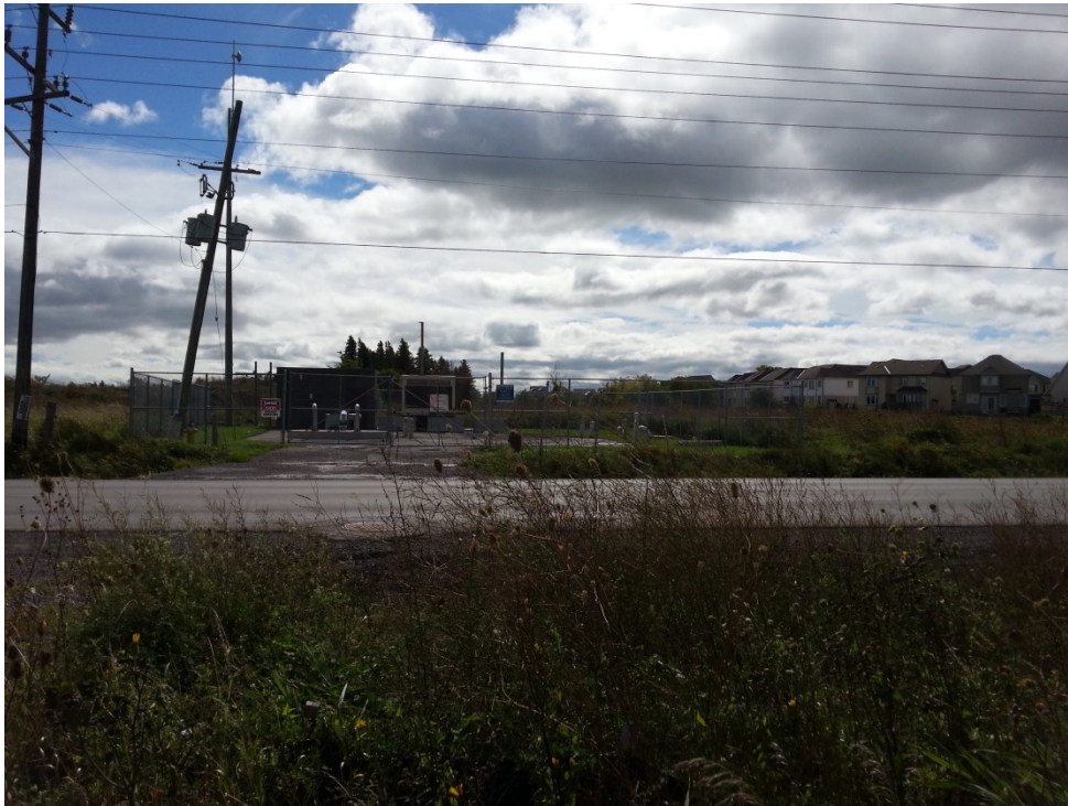
Photograph 3: Looking south at pole mounted transformers and the Maple Grove Road pumping station.
