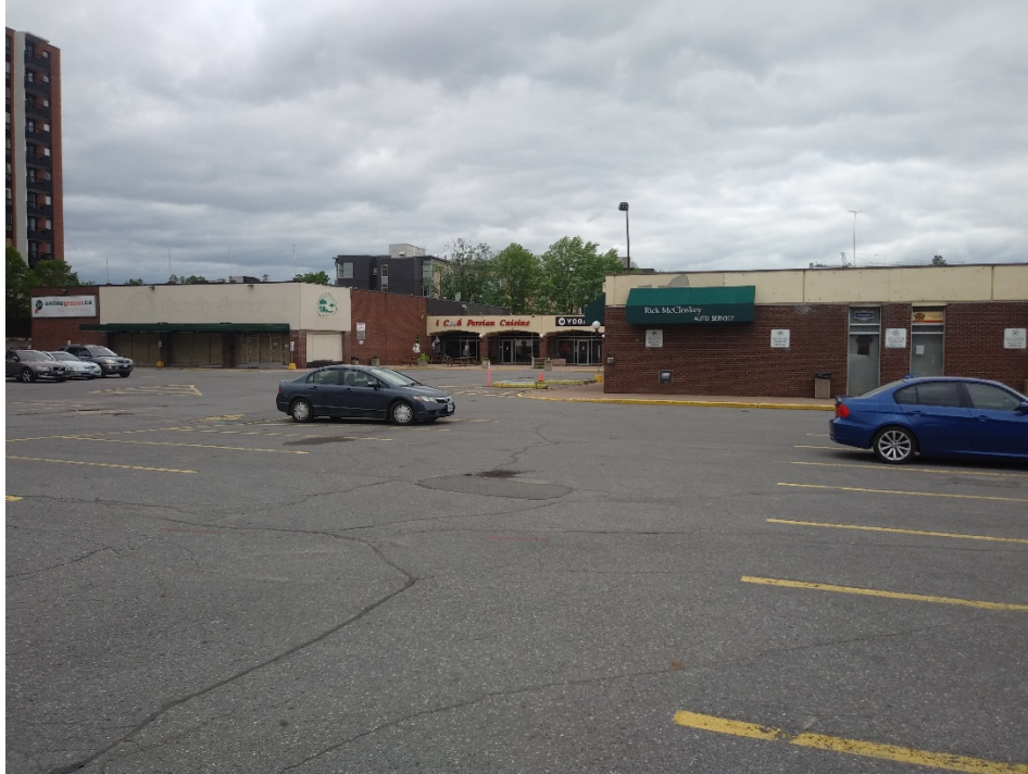
Photograph 1: View of Phase One Property looking north from Ridgewood Drive. View shows the north (right side) and south (left side) commercial buildings at the Property. The automotive service garage is visible in this view.
