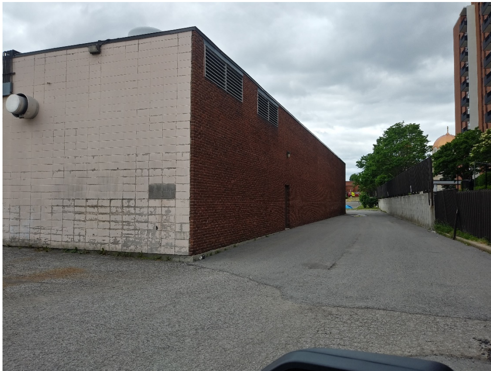
Photograph 4: View of the west side of the Phase One Property looking south. View shows the west side of the north commercial building.
