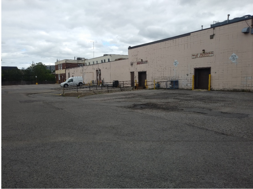
Photograph 3: View of the north side of the Phase One Property looking southeast. View shows the north side of the north commercial building, including the loading dock for the former grocery store and the natural gas meters for the commercial units.
