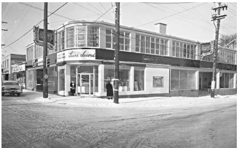
28 Wellington St W and Holland Avenue Junction c. 1955. Urbisite .
