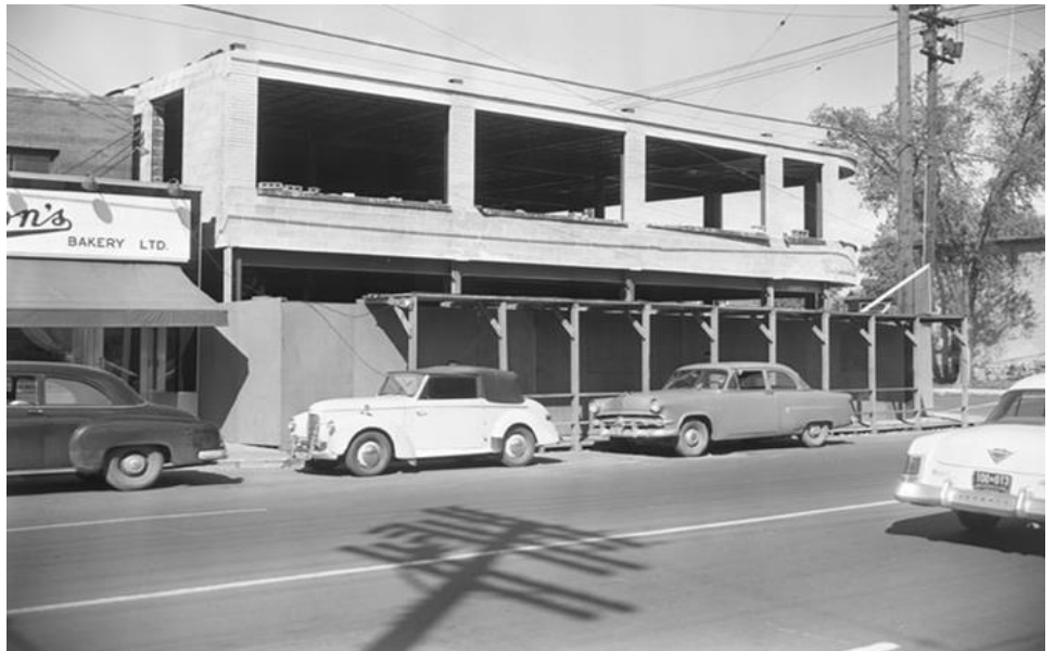
26 1191 Wellington St W, across street from site (now World of Maps), under construction. Kitchissippi Times .
