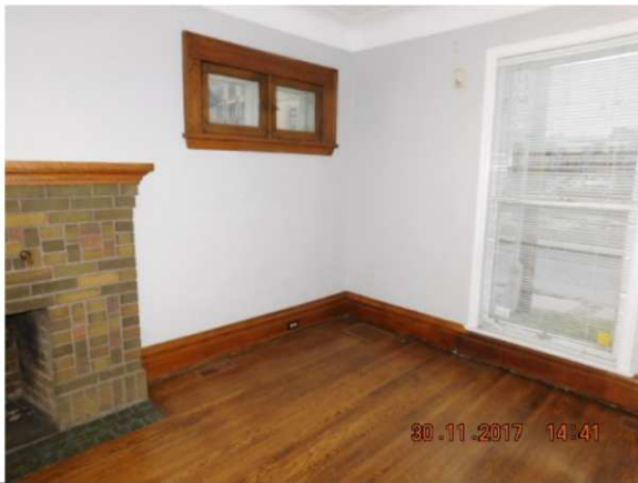
View of the first floor interior. Note the introduced window sill which extends almost to the floor, supporting the theory that the building originally had a more horizontal fenestration pattern similar to 263 McLeod. Note the original window to the right of the fireplace, and the simple casement detailing which is in keeping with a construction date in the 1925 – 30 period. The fireplace brickwork and pattern are also typical of the 1920 – 1930 period.
