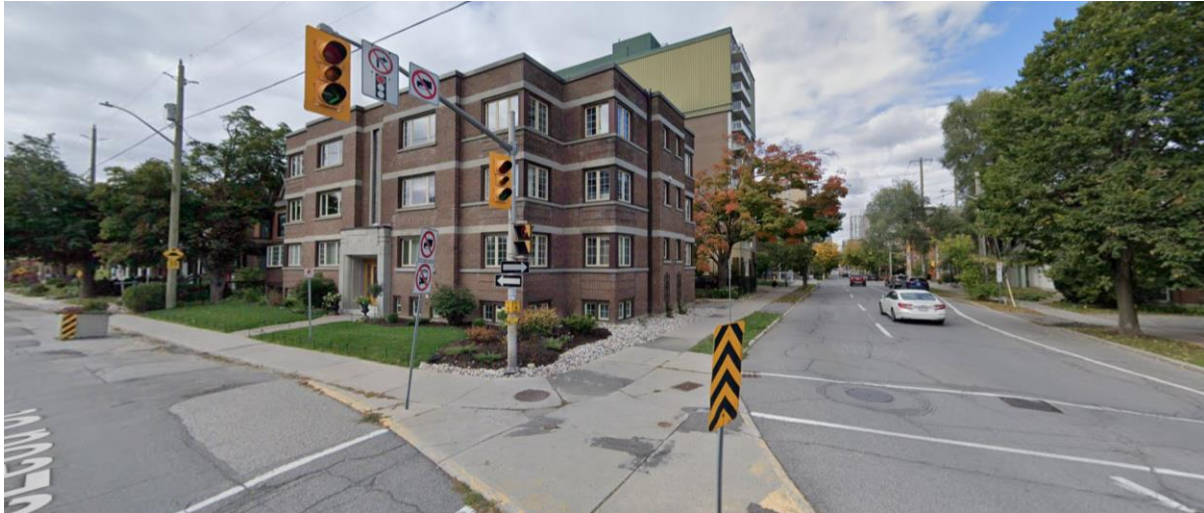
Figure 4: The Appin Apartment at the intersection of Metcalfe and McLeod Streets accents a relatively intact streetscape between O'Connor and Metcalfe. Source Google Maps
