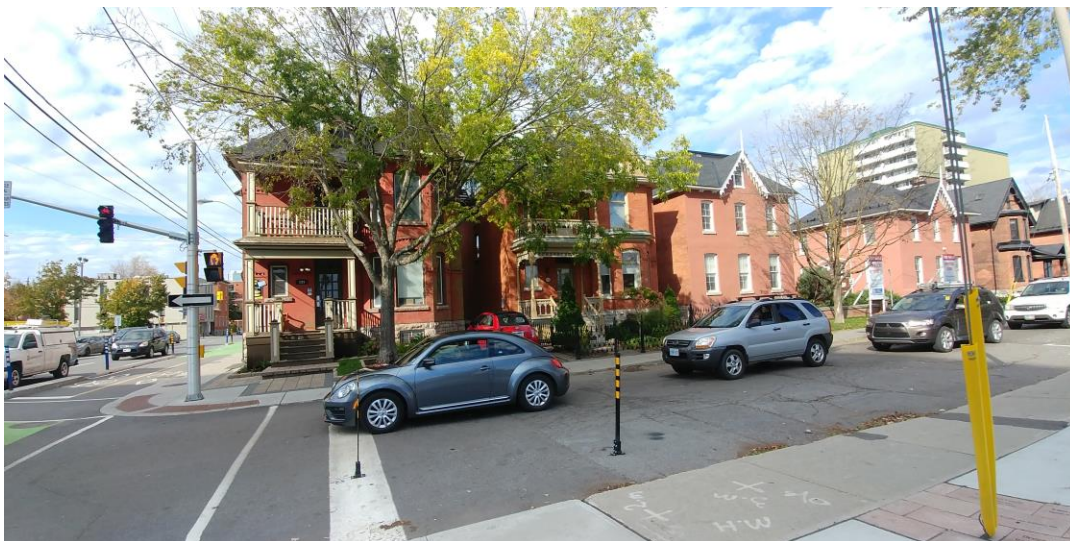
Figure 3: Context view looking north at the intersection of O’Connor. At O’Connor, the grouping of two identical buildings define that corner. The third building in this grouping 385 McLeod was altered. The 12-storey high-rise framing the block at O’Connor and Gladstone is very visible. The 8-storey unit directly behind the subject property is not intrusive from this view. Source: Google Maps
