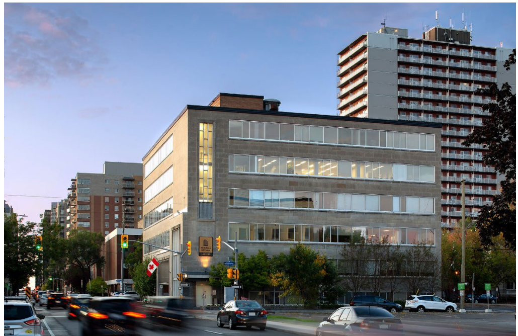
Figure 2.0 – Existing Legion Building at 359 Kent Street.
