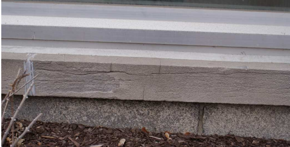
Figure 20: View of a deteriorated limestone windowsill and the granite plinth course below. The cleavage planes within the limestone sills are evident where the sawn surface has weathered. The cleavages planes follow the layers of deposition of the sedimentary rock. Source: Commonwealth 2022.
