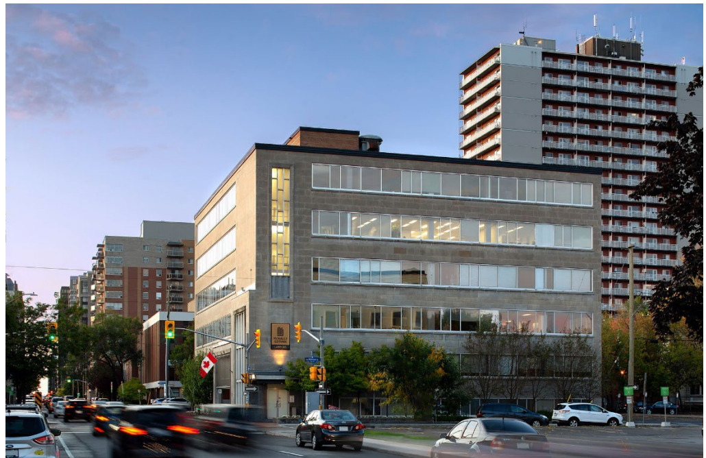
Figure 2.0 – Existing Legion Building at 359 Kent Street.
