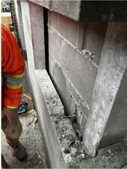
Figure 6: View of a test removal panel from a building at 100 Argyle constructed circa 1955 using a similar limestone cladding material as 359 Kent. The limestone cladding units are secured to the concrete block back-up wall with a single metal anchor centred on the width of the panel. Source: Heritage Grade Test Removal Report, 100 Argyle.
