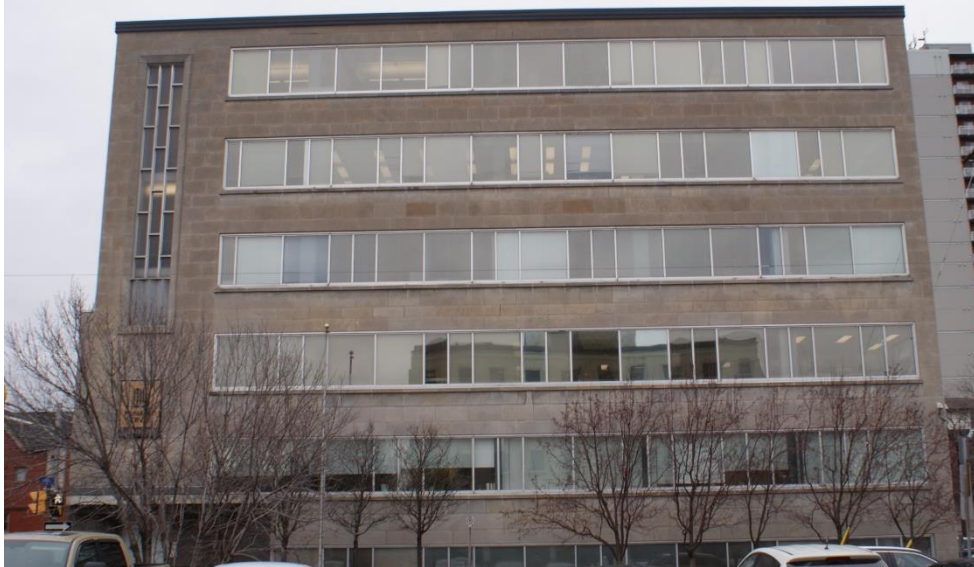
Figure 23: View of the windows on the Gilmour Street façade. All of the original windows have been replaced with the exception of the three-storey window above the Gilmour Street entrance. Source: Commonwealth 2022.
