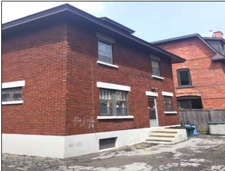
Photo 2 – Site Building (south elevation).
