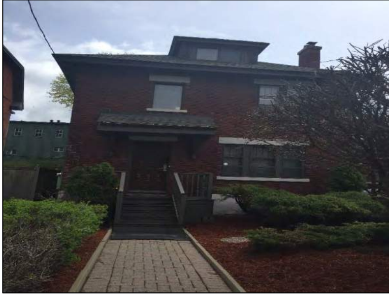
Photo 1 – Site Building (north elevation).
