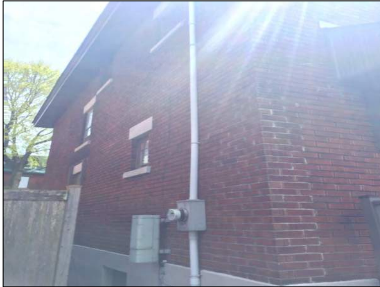
Photo 3 – Site Building (east elevation).
