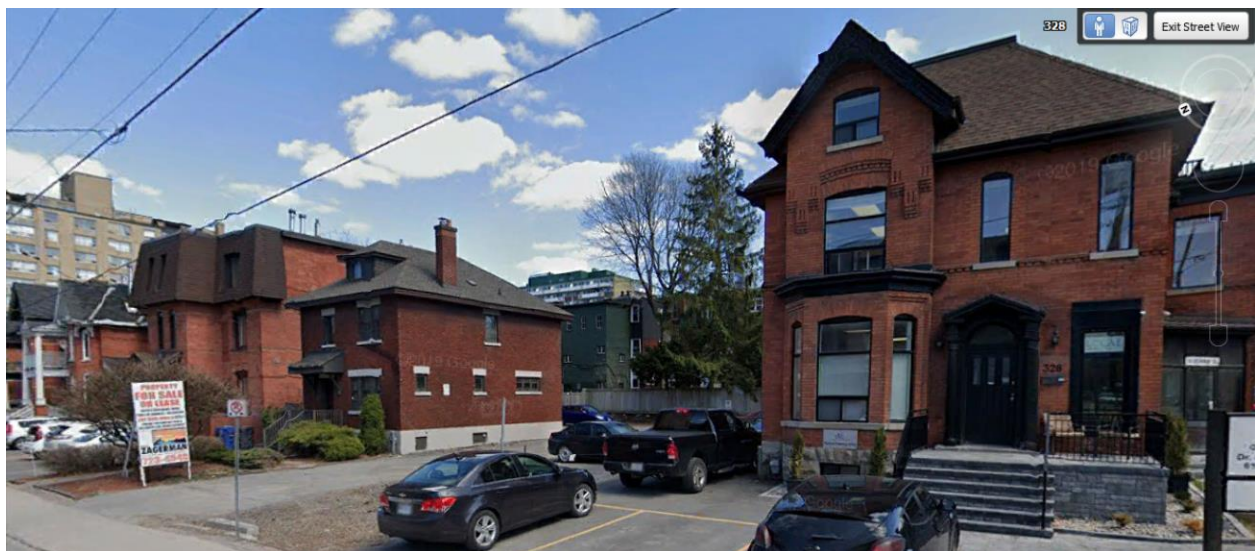
Figure 4: Contextual streetscape view of the development site (322 Waverley centre) illustrating the uniform setback from the street and existing landscape conditions within the lot. The apartment building in the background is one of a number of larger buildings that compromise the neighbourhood. The vacant side-yard visually reads as a gap in the street which is particularly noticeable with the gap mirrored across the street. Source: Google Earth
