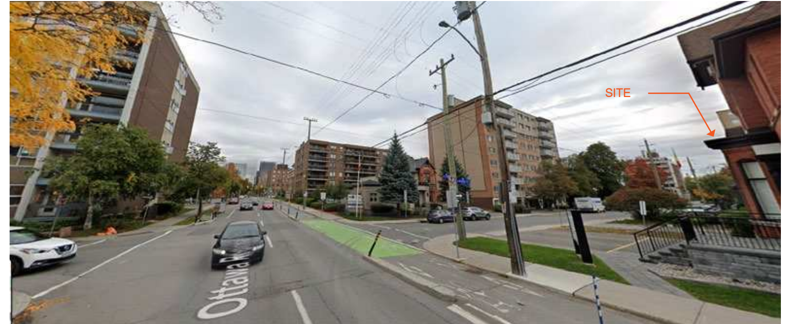
6 - VIEW FROM O'CONNOR ST. LOOKING NORTH-WEST
