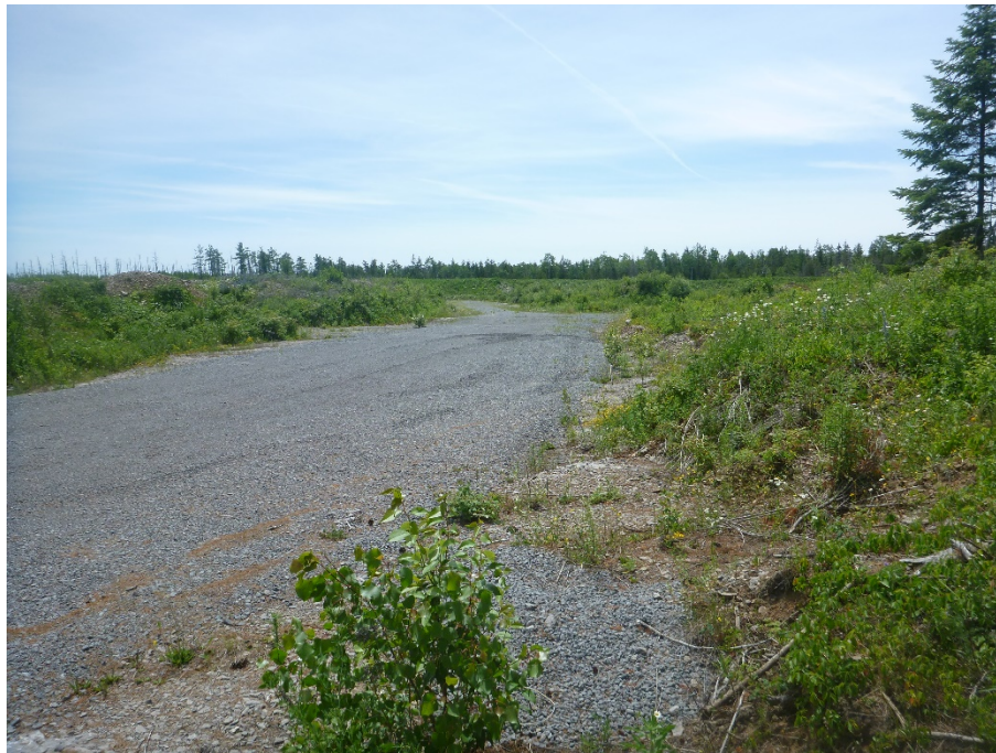
Image 9: Disturbed area showing gravel roadway and large berms facing west.
