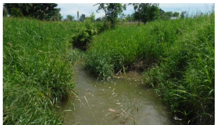
Section downstream of Hwy 417 with high levels of undercutting
