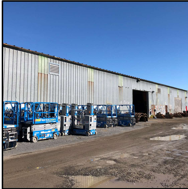
Photograph 1: View of subject building looking north.
