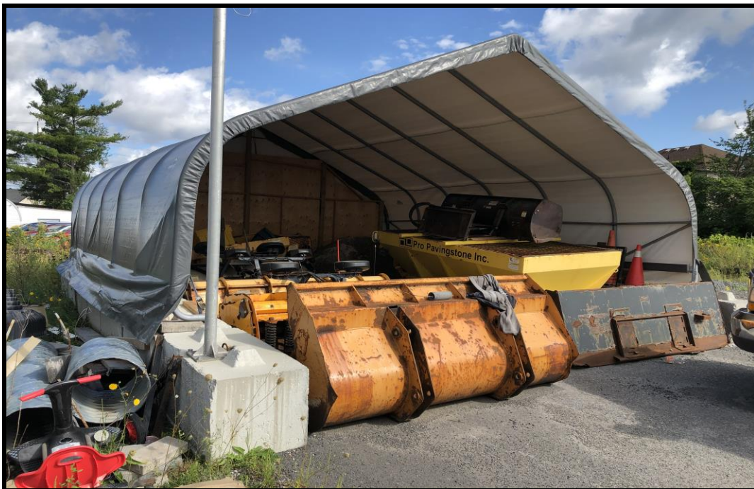
Photograph 4: View of a road salt storage tent, located within the central yard of 1470 Hunt Club Road.
