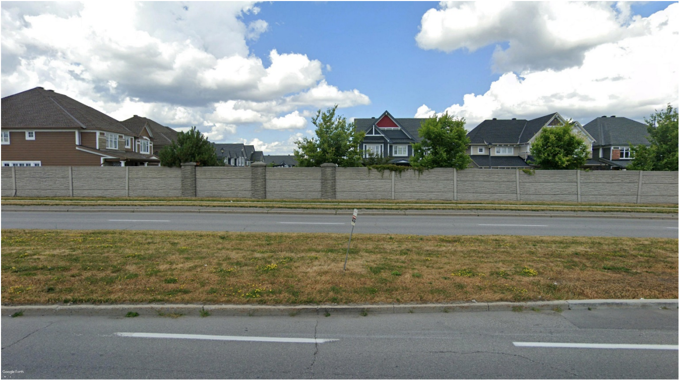
Figure 3: View Looking North (from Hunt Club Road), Across from Subject Property
