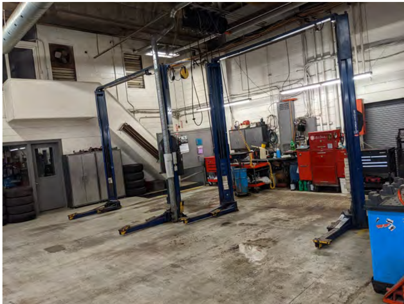
Photo 18 - Hoists in the garage, along westside
