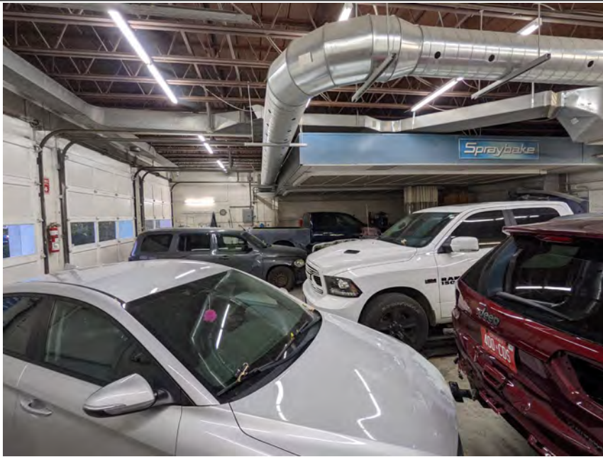
Photo 31 – Interior of the body shop, westside of the building
