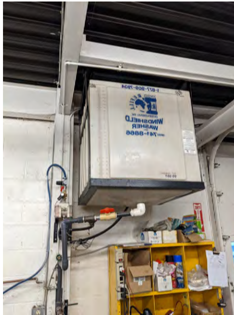
Photo 13 – Washer fluid tote suspended inside the building
