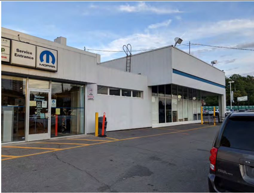
Photo 3 – West side of the building, looking north
