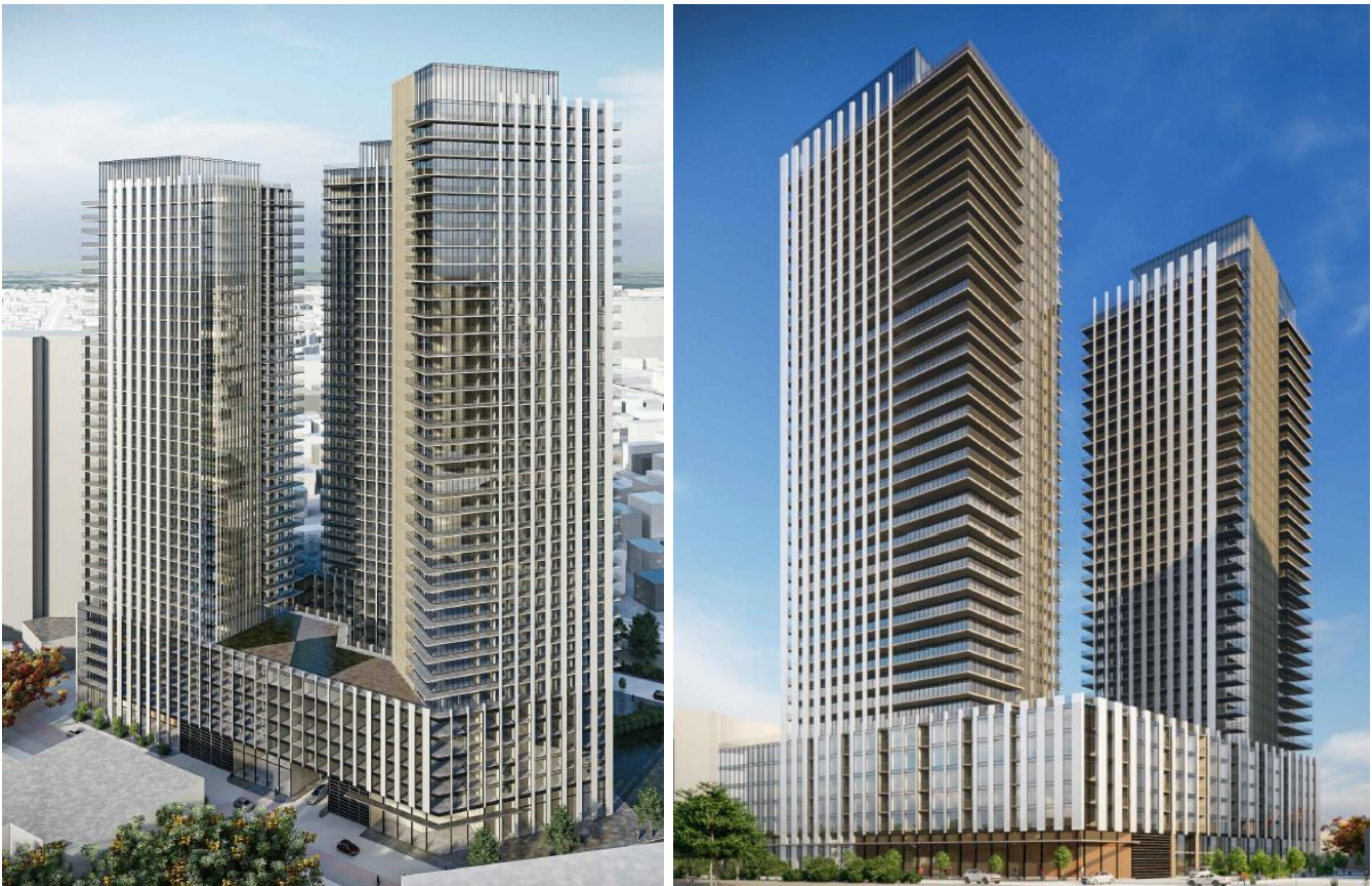
Figure 8: Looking southeast and northwest towards subject site
