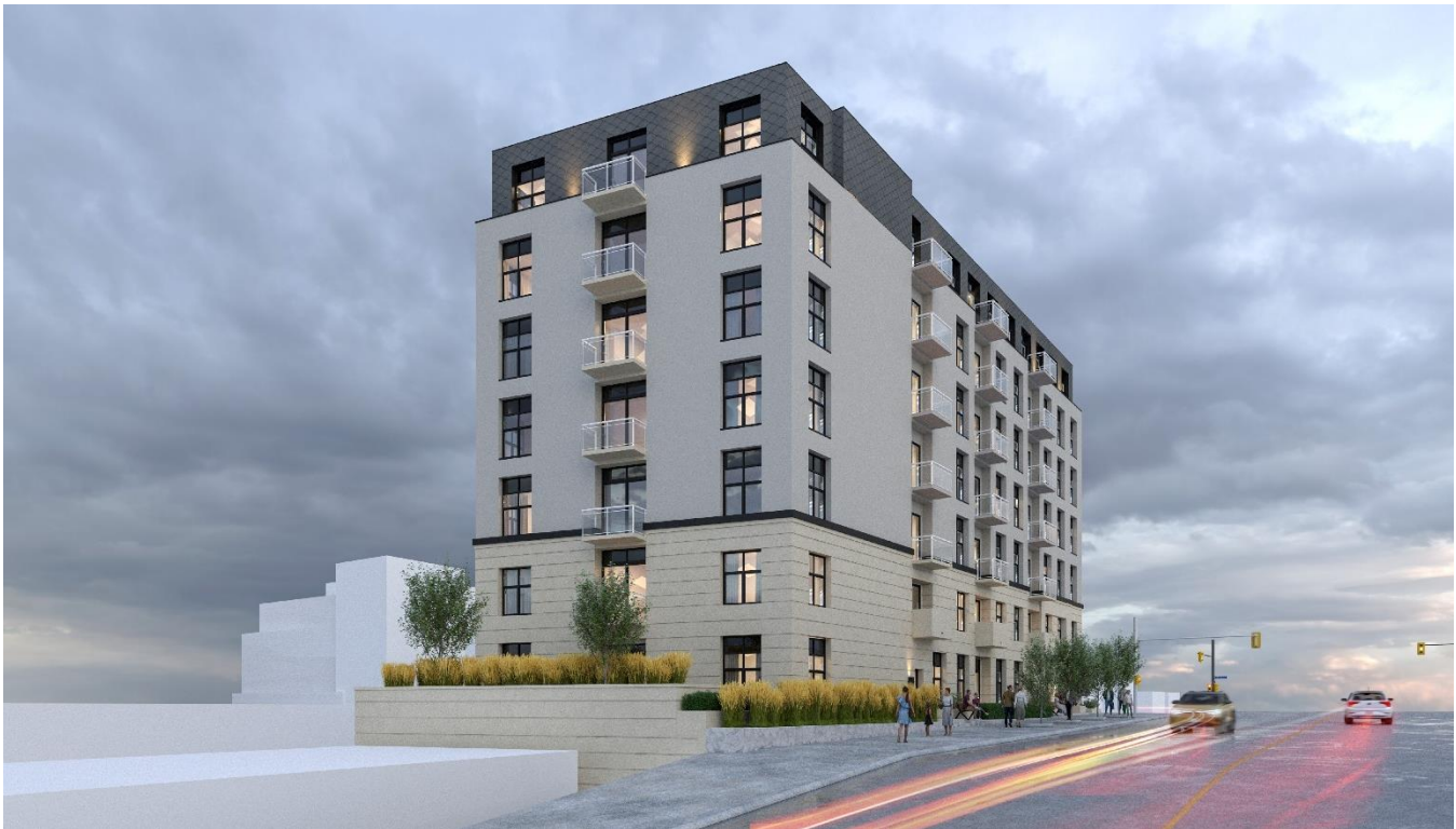
Figure 16: Building materiality from Byron Avenue, looking east towards Churchill Avenue North
