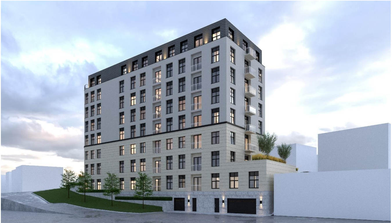
Figure 19: Pedestrian level view of parking garage on Danforth Avenue looking east towards Churchill Avenue North
