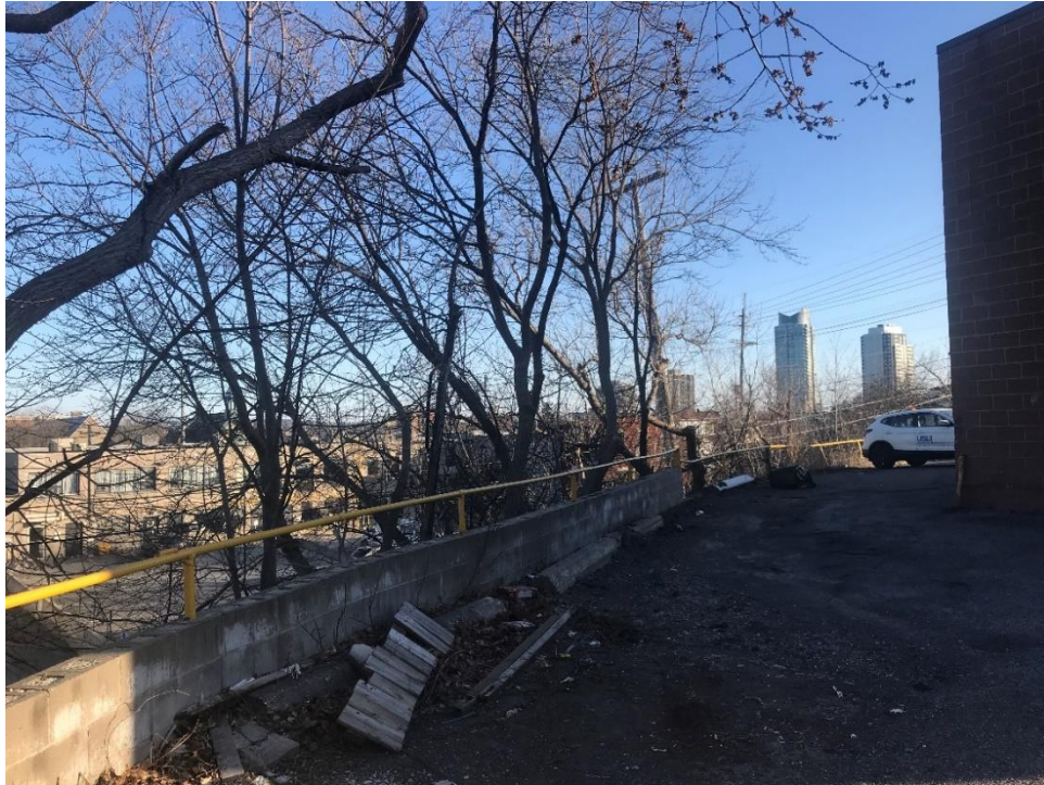
Photograph 7: West perimeter of Site, facing north (April 6, 2021).
