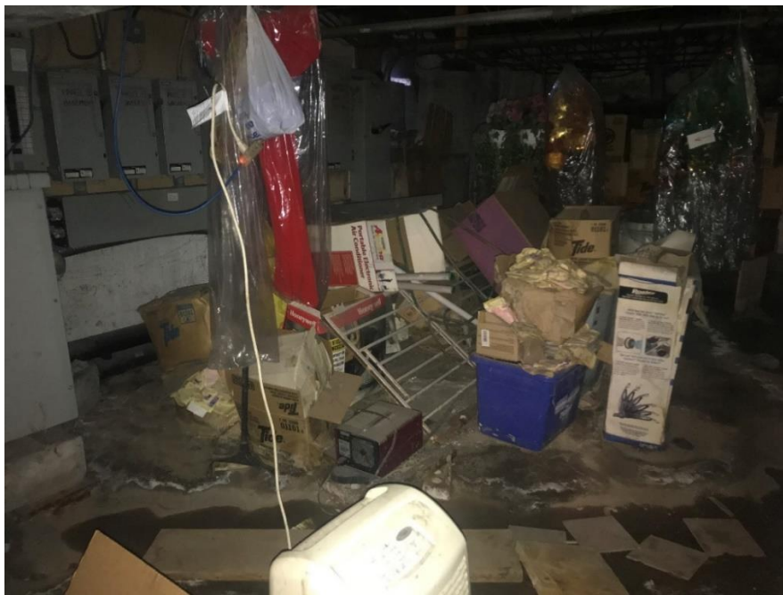
Photograph 26: Site building basement, storage (April 6, 2021).
