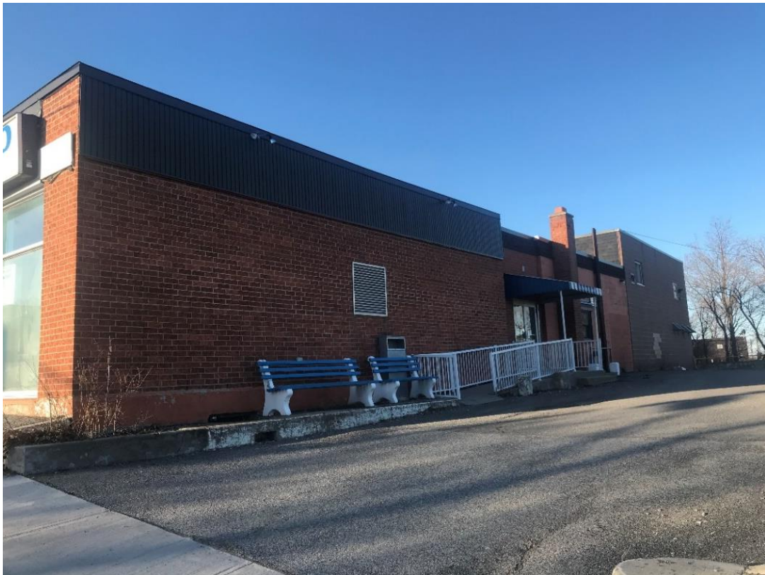
Photograph 2: Northeast face of Site building, facing southwest (April 6, 2021).
