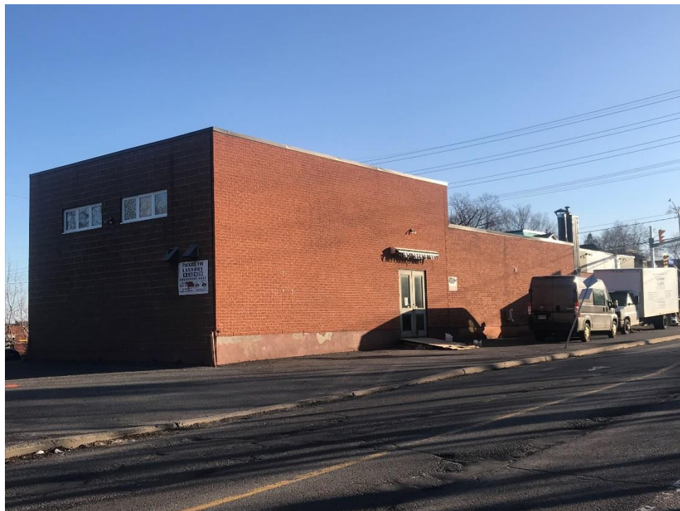
Photograph 8: Southwest face of Site building, facing northeast (April 6, 2021).
