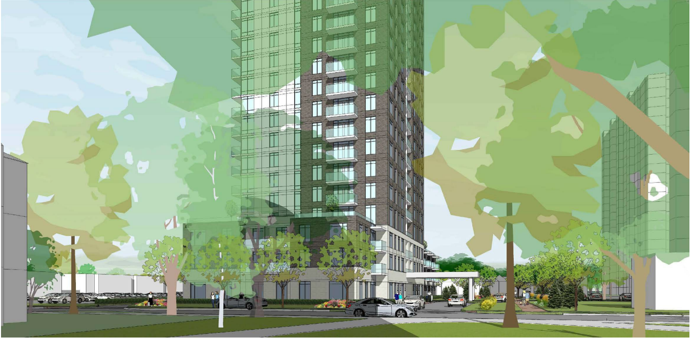
Figure 17. View of the Proposed Development from the South (Lanark Avenue)
