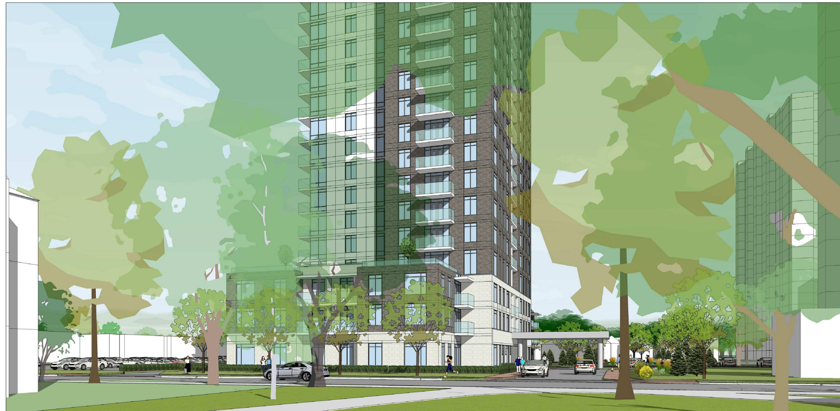
LOOKING NORTHEAST TOWARD THE BUILDING ENTRANCE
