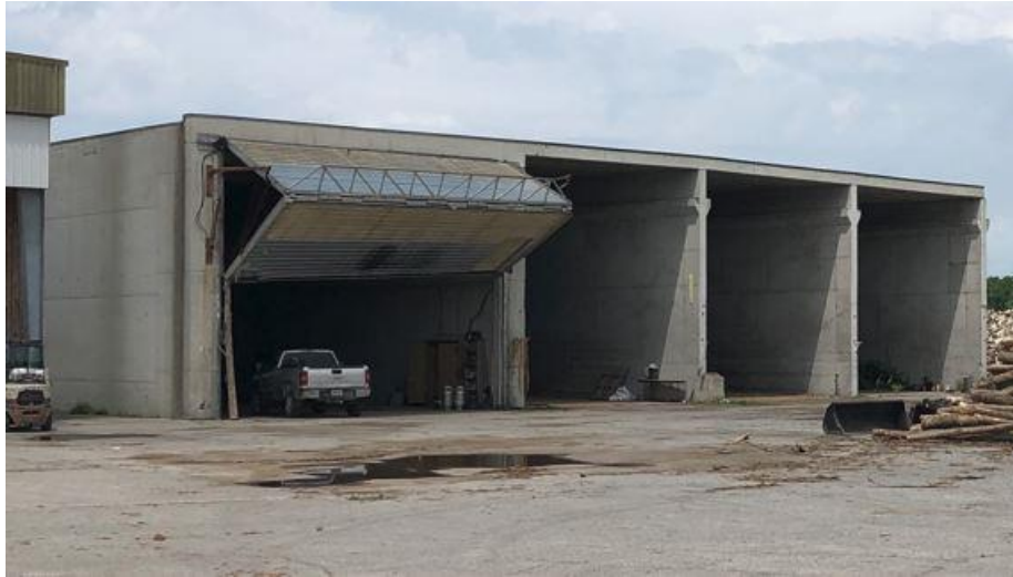
Figure 11 – Concrete Storage Bunker On-Site
