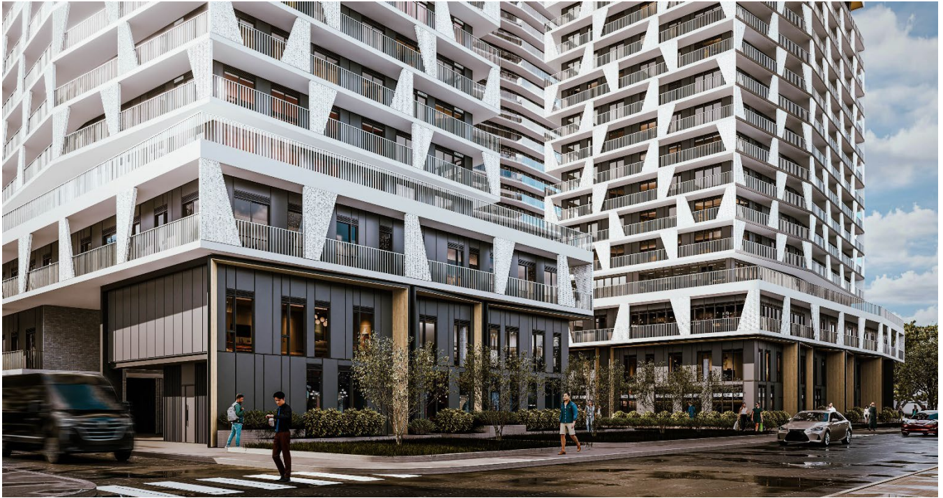
Figure 33. View of the proposed development looking southwest on Brisebois Crescent
