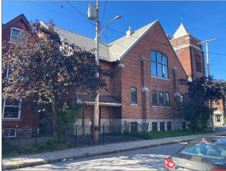
Photo 1 – Site Building (north elevation).
