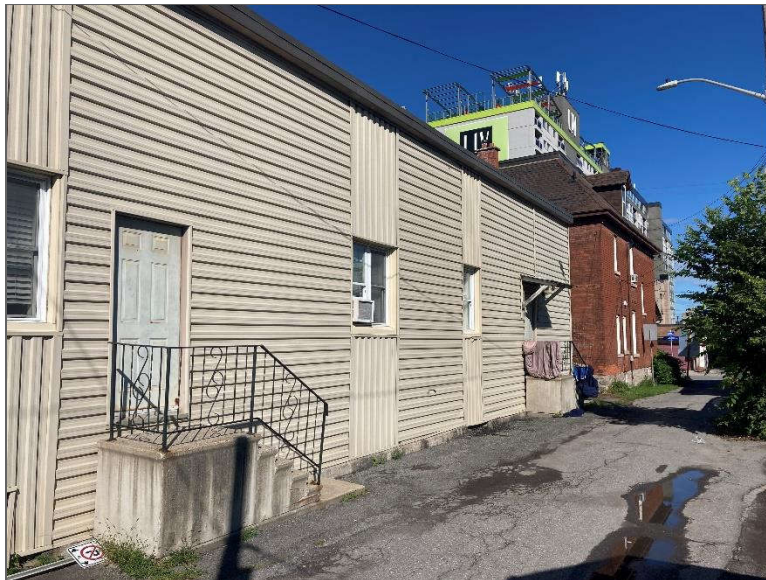
Photo 2 – Site Building (east elevation).
