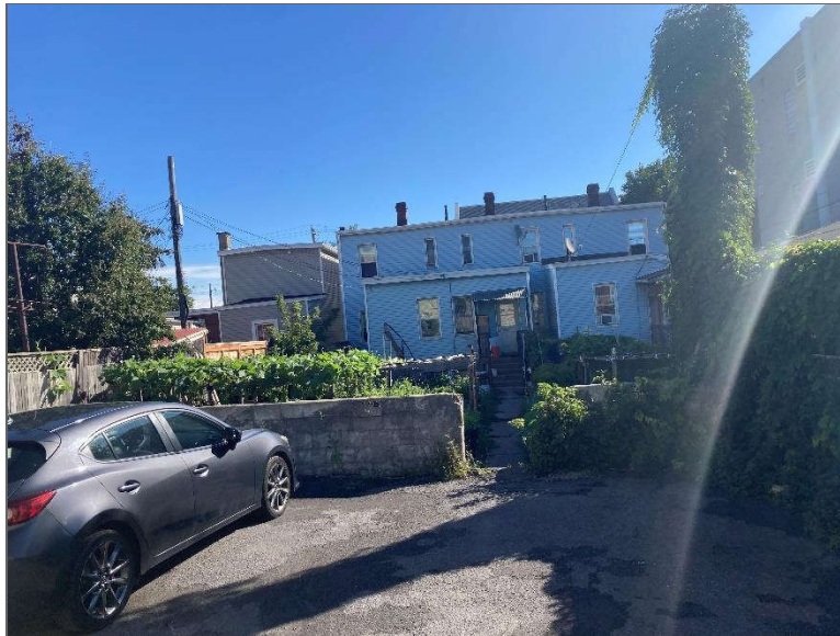
Photo 6 – Properties located east of the Phase One Property.
