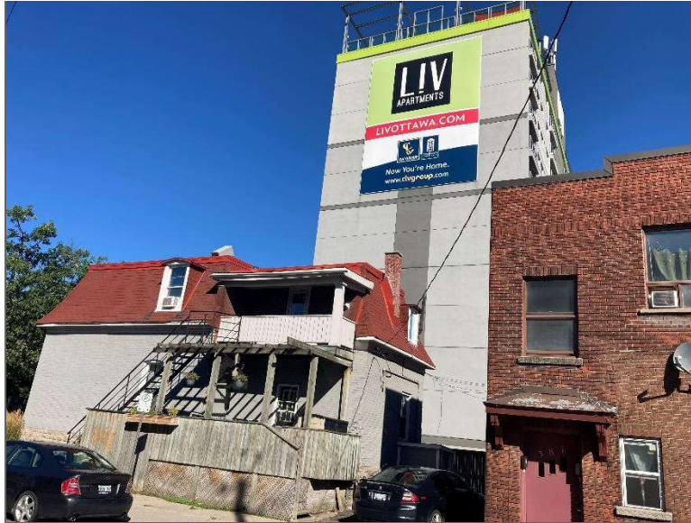
Photo 5 – Properties located north of the Phase One Property.
