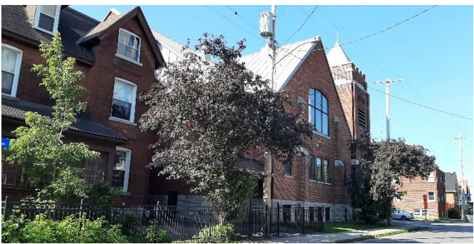
Figure 1: The walls of the north and west façade of the church, shown in the right of the photo, are proposed to be retained and the two (2) storey brick dwelling to the east of the church, shown in the left of the photo, is proposed to be demolished
