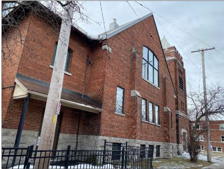
Photo 1 – Site Building (north elevation).
