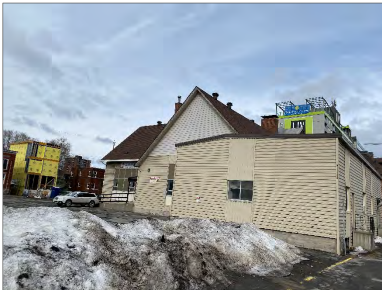
Photo 2 – Site Building (south elevation).
