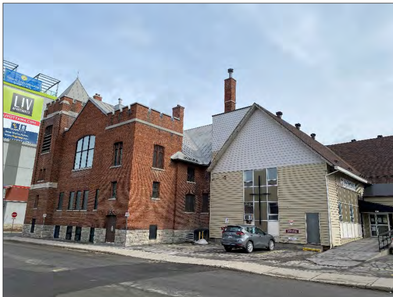
Photo 4 – Site Building (west elevation).
