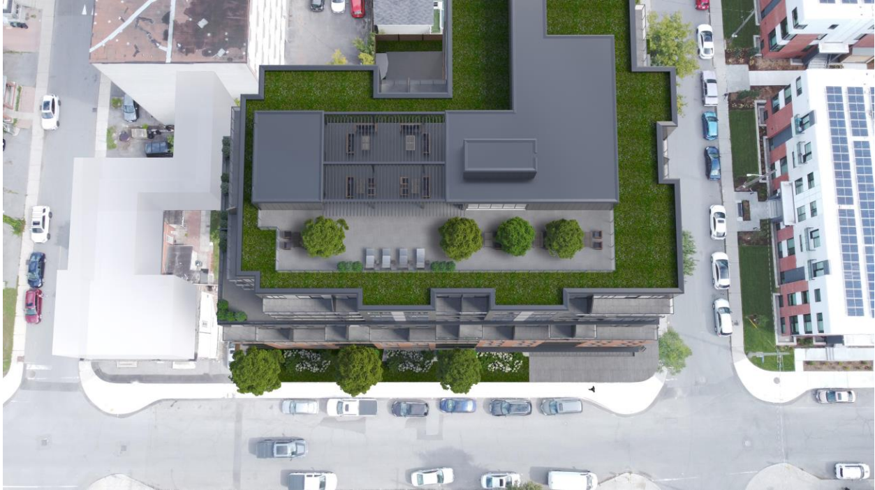
Figure 47: Aerial View of Rooftop Terrace
