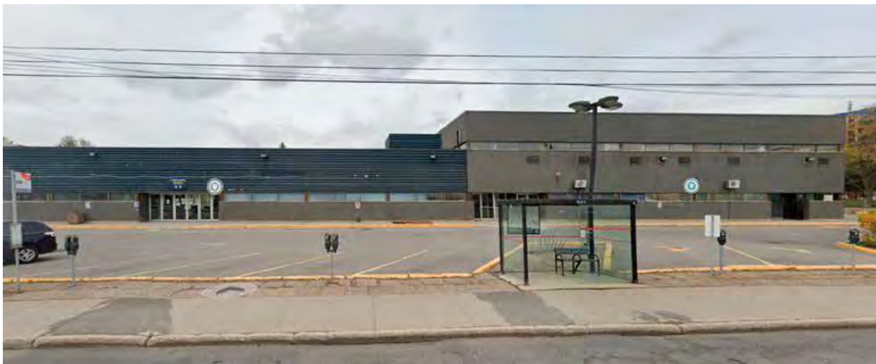
Figure 1 – Former Ottawa Bus Depot (Catherine Street Elevation)
