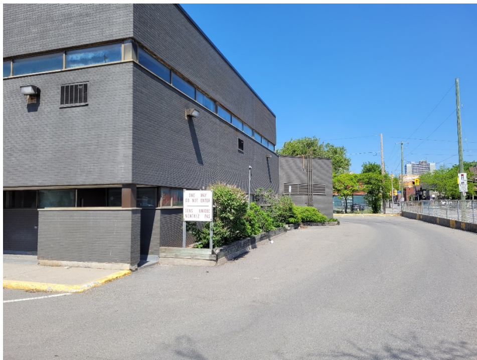
Photograph 2: View of Phase One Property looking north from the southeast corner of the Property. View shows the vent pipes associate with a former aboveground fuel storage tank and an underground waste oil storage tank, associated with the service garage on the east portion of the Property.
