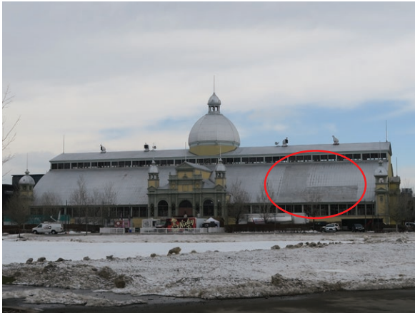
South lower roof. Note fabric covering (ERA 2023)
