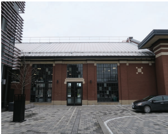
Standing seam metal roof on west elevation (ERA 2023)
