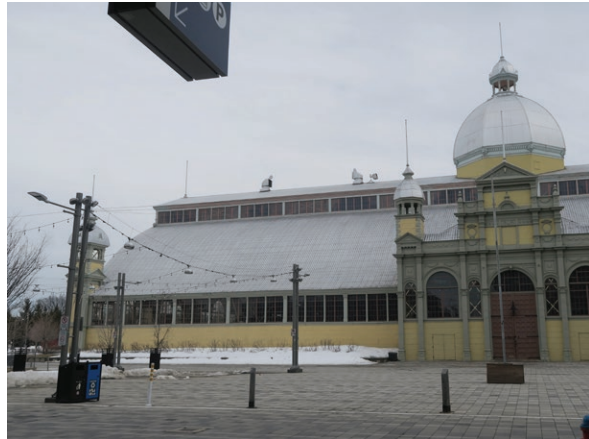
North upper roof: east section. (ERA 2023)
