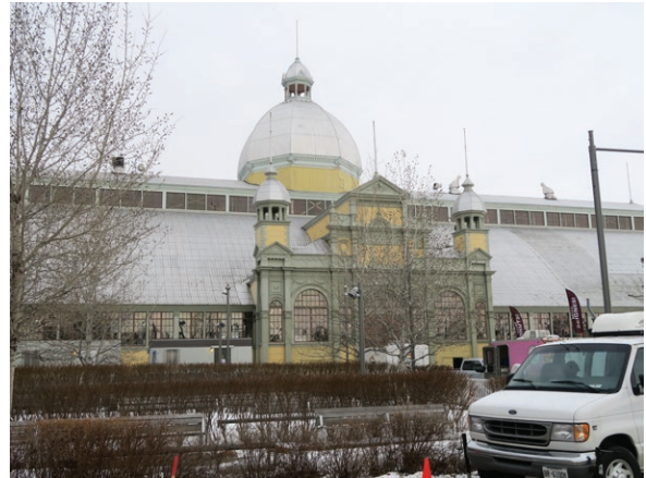
South elevation entrance pavilion (ERA 2023)
