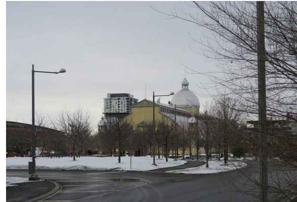
Looking west from Princess Patricia Way towards the Aberdeen Pavilion (ERA, 2023).
