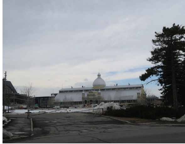
Looking northwest from the Site's Queen Elizabeth Driveway service entrance. The Aberdeen Pavilion is at the centre (ERA, 2023).
