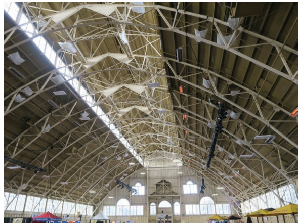
Interior underside of roof: looking west (ERA 2019)
