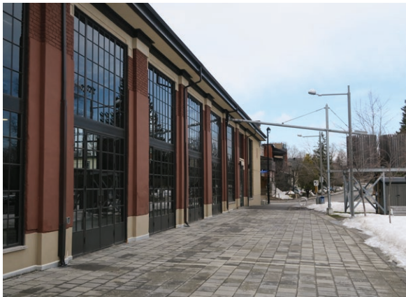
Metal doors on the east elevation of the exhibition hall (ERA 2023)
