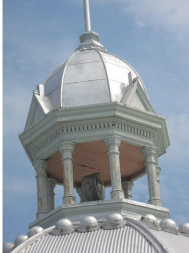
Roof cupola from south (ERA 2019)
