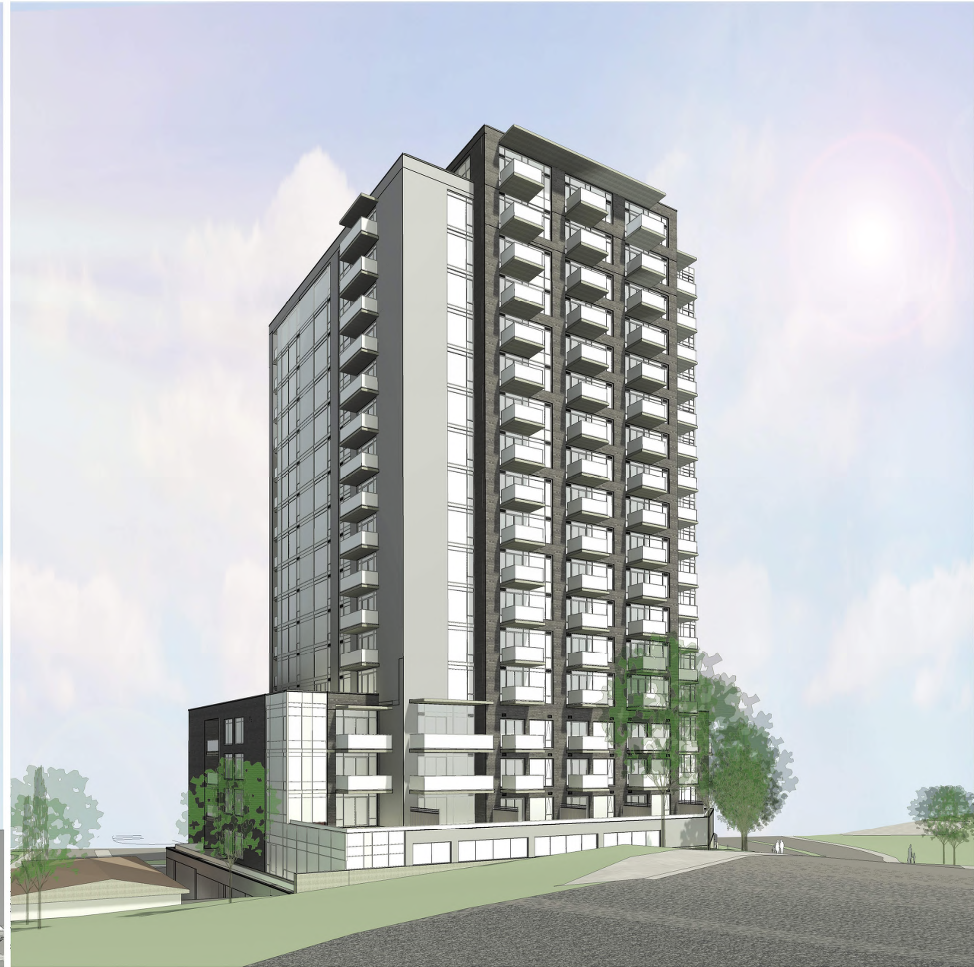
VIEW LOOKING NORTH EAST FROM DUFORD DRIVE
