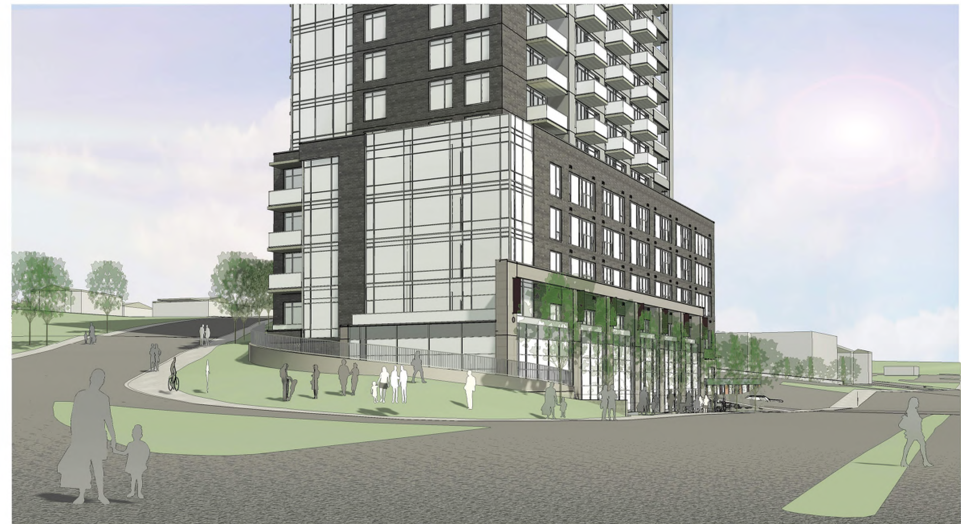
ENLARGED VIEW LOOKING WEST AT PODIUM
