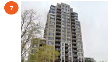
7 75 CLEARY AVE. 16-STOUREY RESIDENTIAL BUILDING
