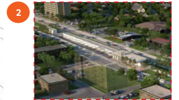
2 FUTURE LRT SHERBOURNE STATION
