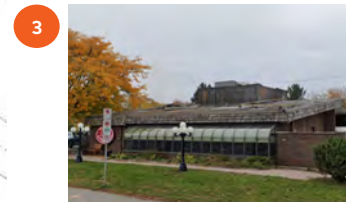
3 809 RICHMOND RD. EXISTING 1-STOUREY RESTAURANT
