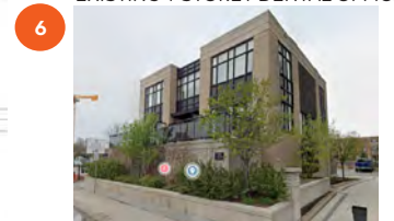
6 773 RICHMOND RD. 3-STOUREY RESIDENTIAL BUILDING
