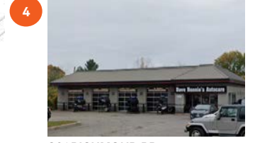
801 RICHMOND RD. EXISTING 1-STORY AUTO SHOP
