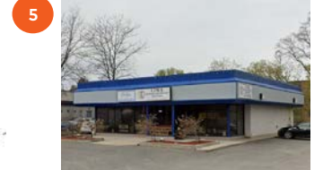
797 RICHMOND RD. EXISTING 1-STORY DENTAL OFFICE
