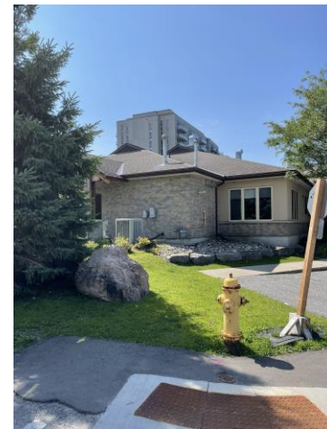
Photo 10 - River Parkway Children's Centre. Taken from Phase One Property, facing southwest
