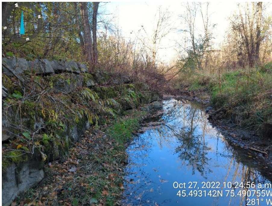
Photo 10: Taylor Creek near the center of its length, looking downstream, retaining wall present (October 27, 2022)
