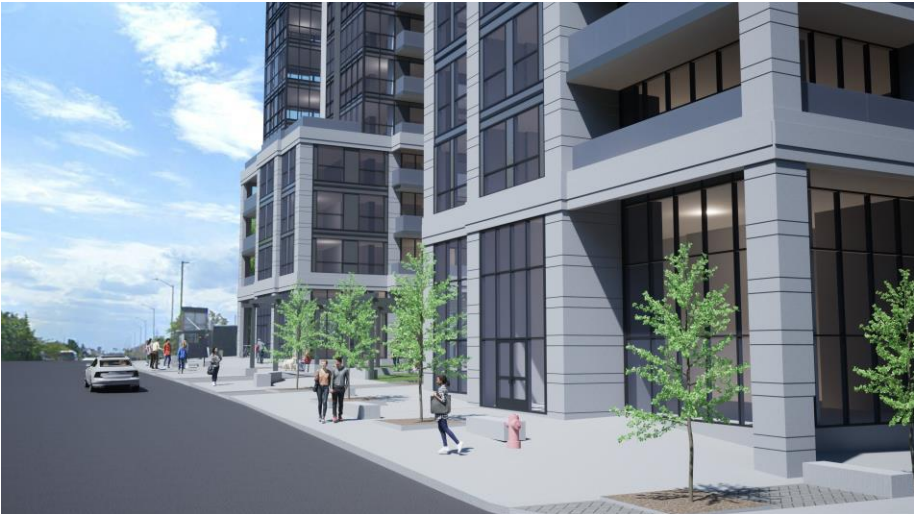
Southeast corner of building on Marketplace Ave.
