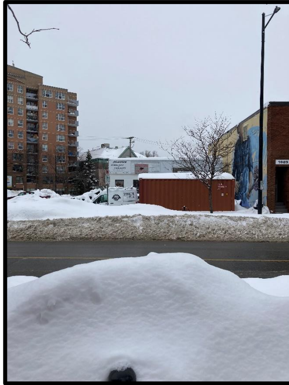
Photograph 7: View of the automotive service garage on the 1 Spadina Avenue property from the northwest corner of the Phase I Property, facing north.
