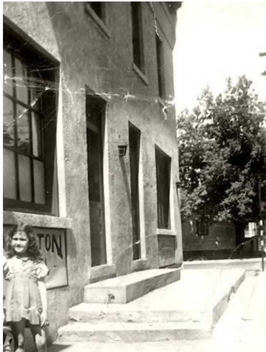
Figure 8: This photo showing the stucco treatment, the large industrial windows on either side of the front entrance with the two-door entry doors from the mid-60s. A later renovation introduced the masonry stone veneer, and leaded-glass windows, with the Tudor treatment to the upper floor and cornice.
