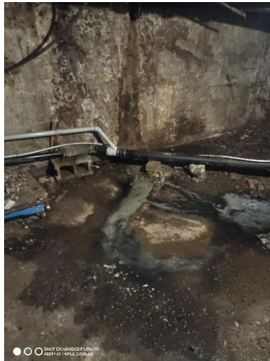
Figures 25: The leaded glass of the front windows is a later addition when a Tudor Style Attributes were introduced. Figure 26 and 27: Two views of the basement crawl space with seepage of groundwater through the native rock. .
