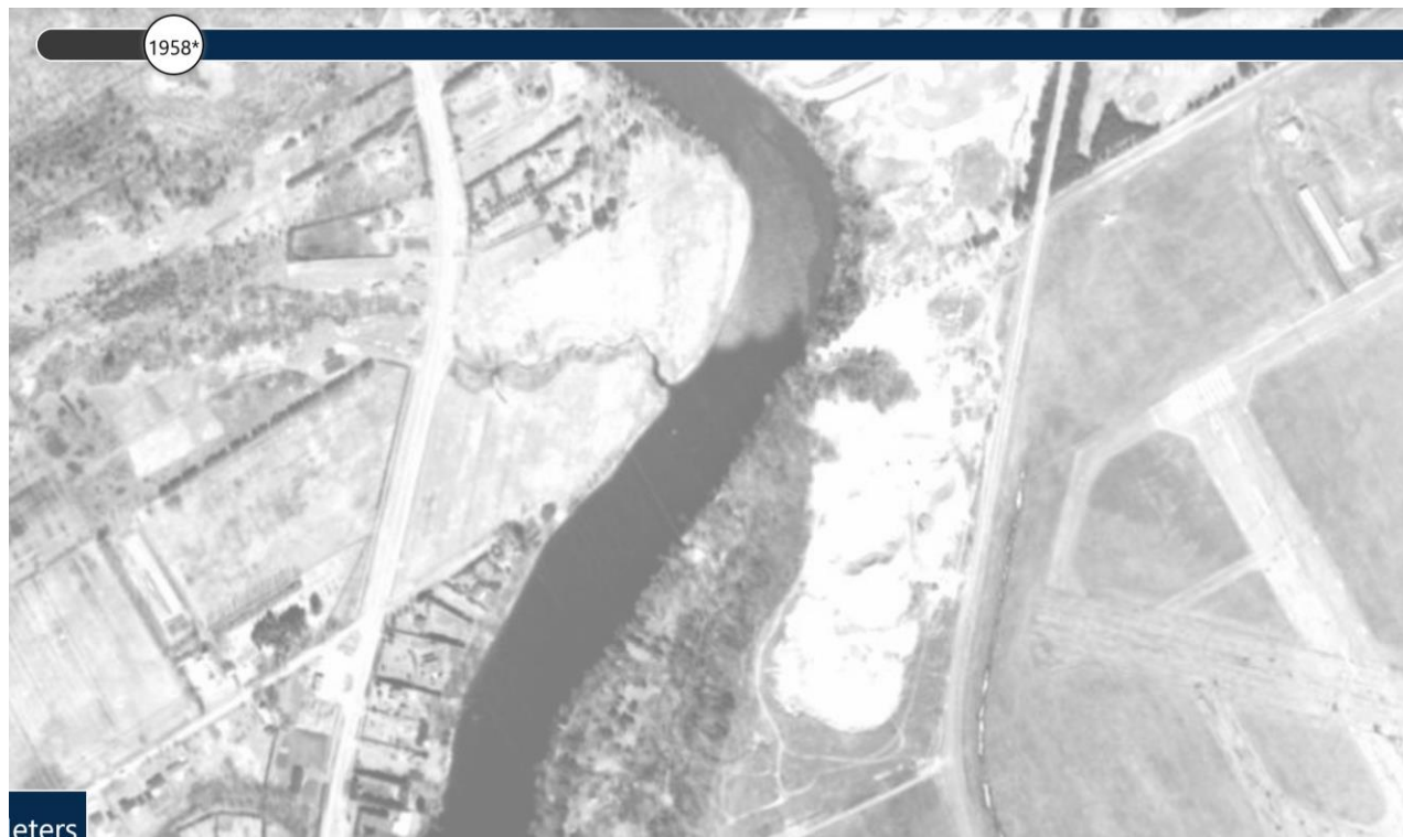
Figure 6: Aerial view 1958 is one of the earliest views prior to the West Hunt Club bridge over the River. Source: Geo Ottawa
