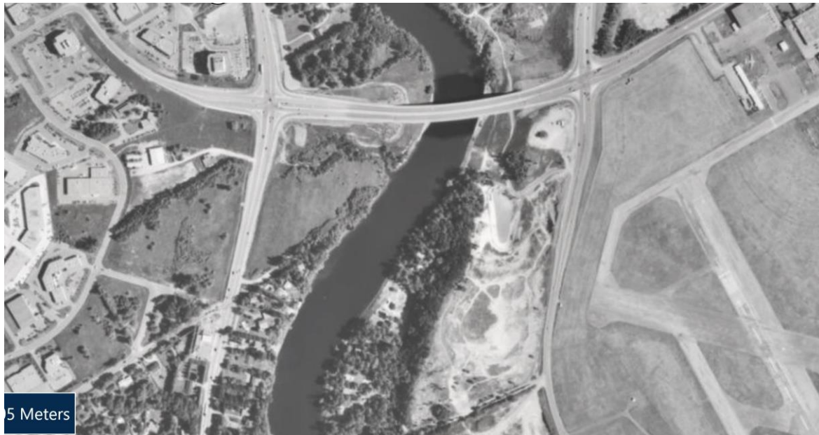
Figure 7: Aerial view 1991 with the bridge in place, the abutment on the east side of the bridge appears as newly installed just north of the tributary ravine. Source: Geo Ottawa
