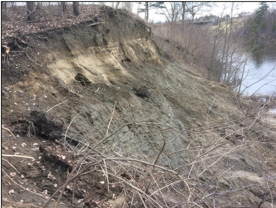
Photo 2: Existing slope conditions along slope located to the southwest of the subject site. Recent slip failure has occurred and left steep backscarp.
