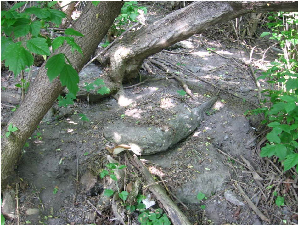
Photo 17. Eroding slope above the shoreline – May 25, 2010.
