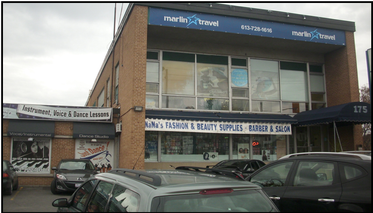
Photograph 2: South wall of eastern portion of the building, facing north.
