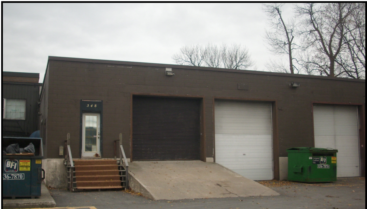
Photograph 4: South wall of the northern portion of the building, facing south.
