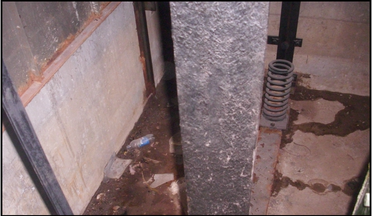
Photograph 5: Floor of elevator pit.
