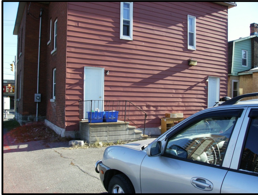
Photograph 3: 250-252 Parkdale Avenue, facing east.
